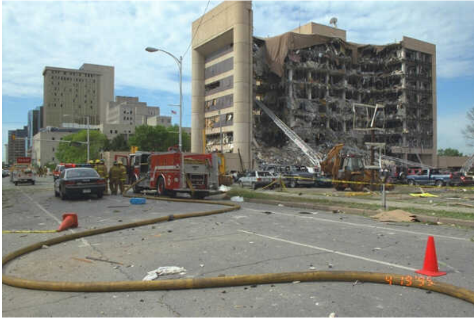
Pic. 2: Alfred P. Murrah Federal Building Bombing, Oklahoma City, Oklahoma, United States, April 19, 1995
